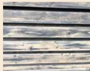
Visible treatment solution drying marks
