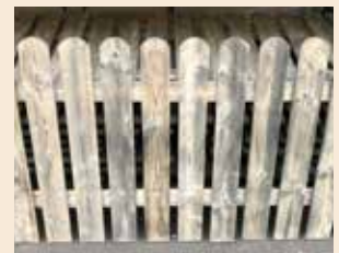
Visible treatment solution drying marks
